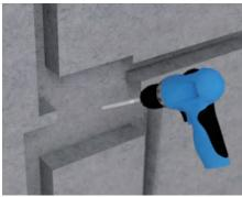
2、The depth of the embedded box is 1.8"-2.4". It's better to drill the depth of 1.8"for blank wall.
